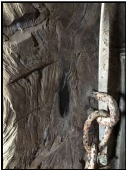
Right, burn marks in the stables at Sherwood, Hollow Tree, Tasmania.
